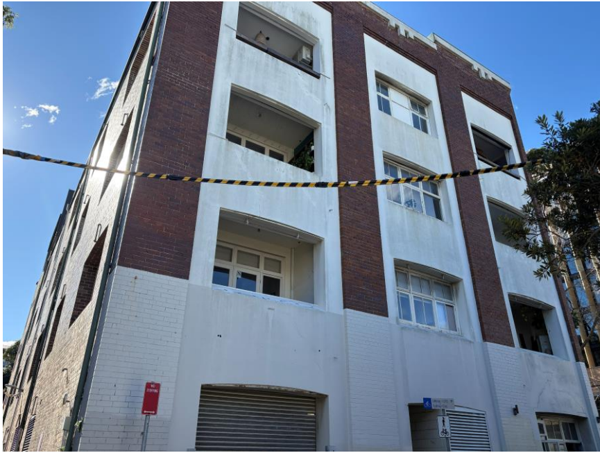
Figure 1: 27-39 Abercrombie Street, Chippendale viewed from the north-west
